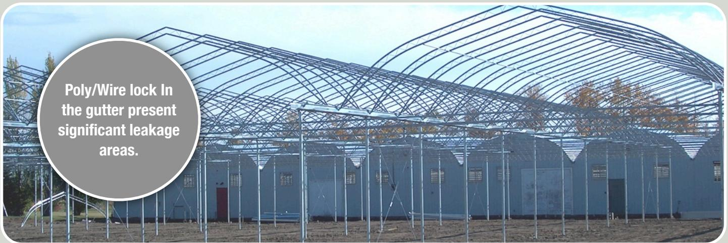
Poly/Wire lock In the gutter present significant leakage areas.
